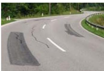
**Bituminous asphalt sealer** used for crack repair is extremely slick, especially when wet, and is well known for causing motorcycle accidents. Alternative repair methods exist and should be adopted. Further research and a review of standards (EN 1423) are needed. A replacement for existing bituminous asphalt sealer such as the cold-setting Austrian product Stohflex which retains high frictional properties when subject to wear is recommended.
